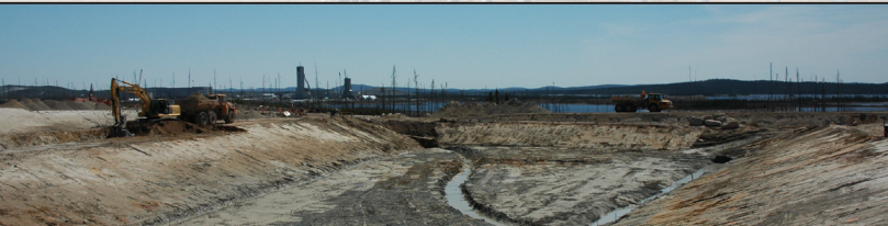
Making of used water treatment basins
