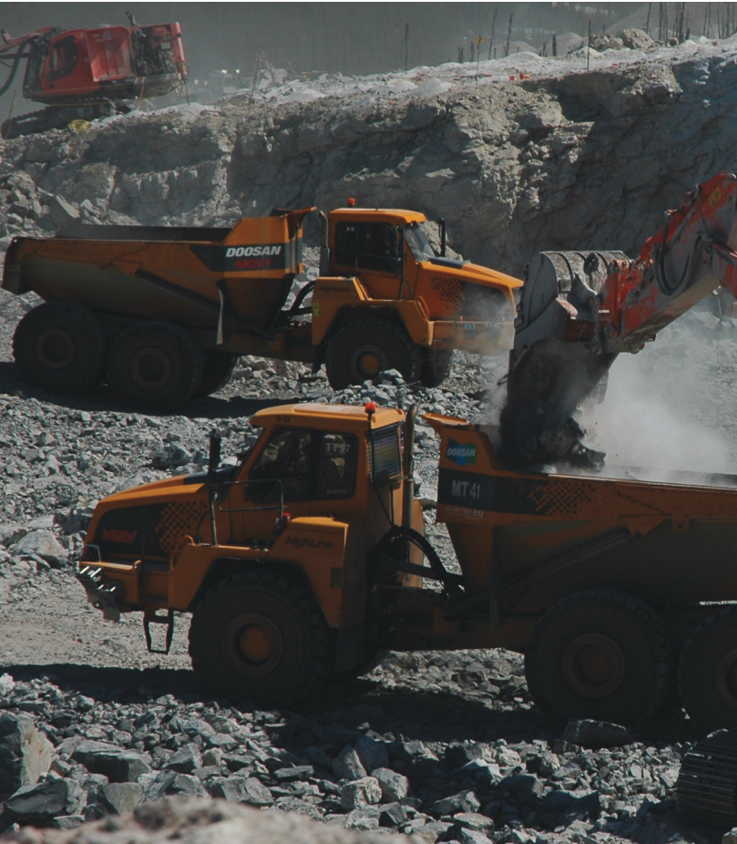
Rock excavation in a pit for production of aggregates
