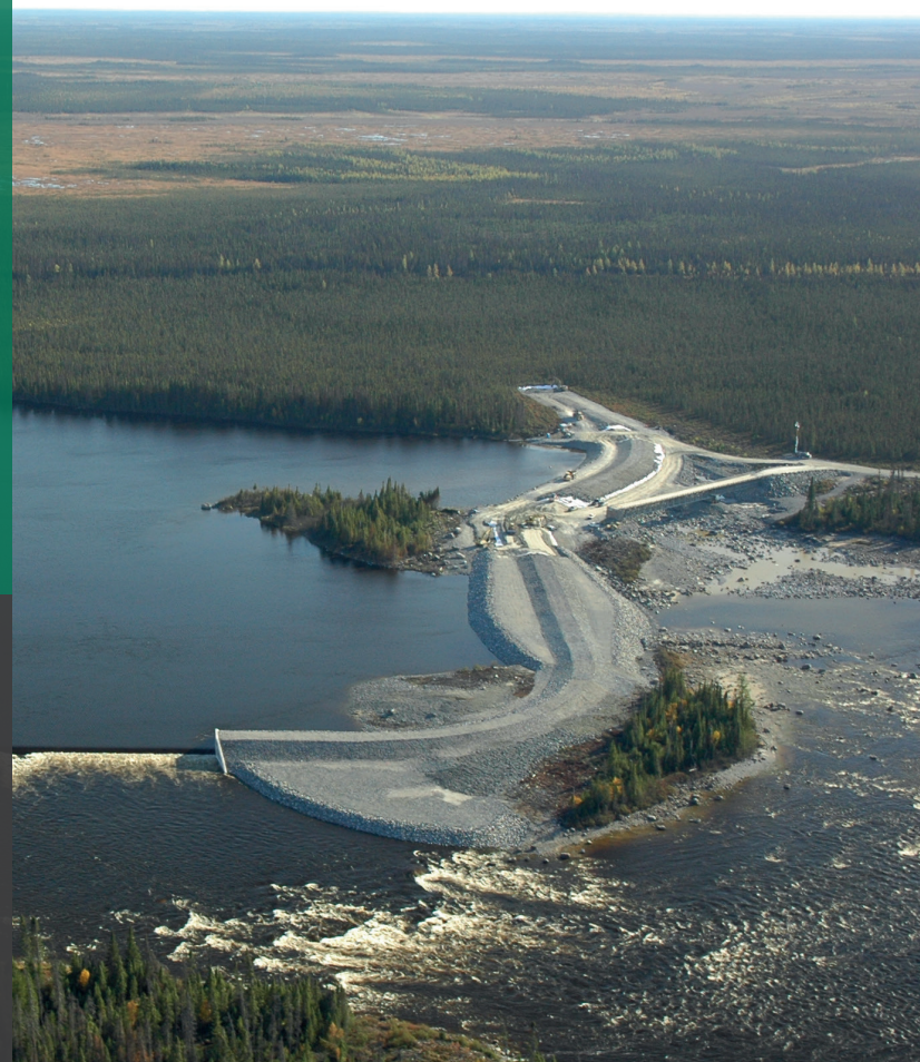
Weir at KP 33 (partial underwater concreting)
