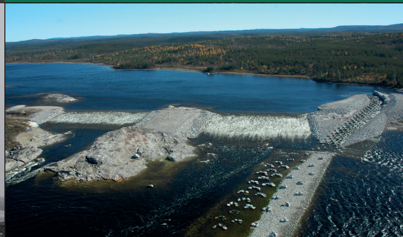
Weir at KP 290 with fish pass
