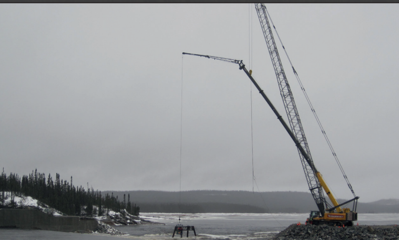
Removal of Bailey bridge piles
